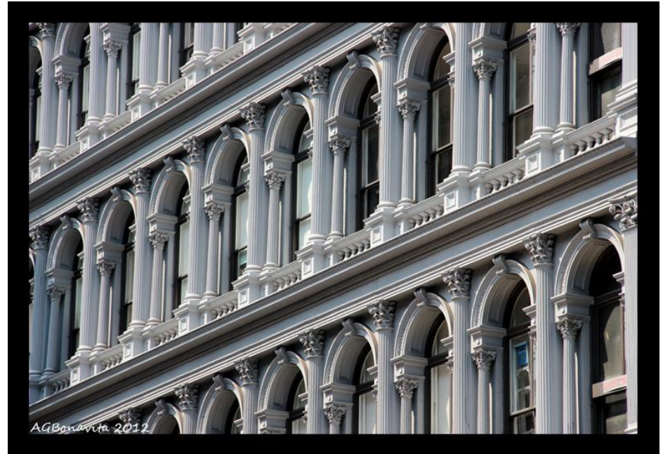
New York's Haughwout Building(1857)
